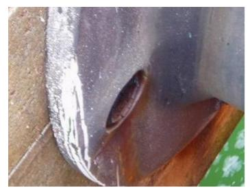
Photo 2.3.11 Missing fixing bolt
