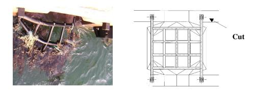
Photo 3.6.2 Example (f cut on flange of Rubber net-Deterioration score"6 points"
