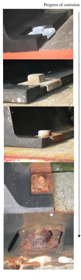
Photo D-2 Example of deterioration rank (Corrosion)
