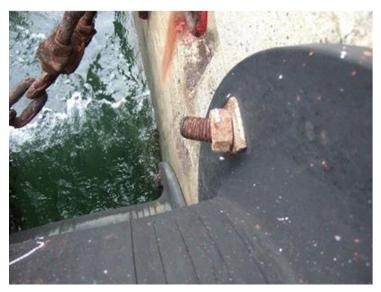
Photo 2.3.10 Bent fixing bolt
