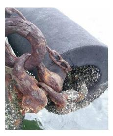
Photo 2.5.4 Corrosion of support
