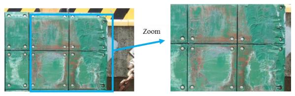
Photo 2.3.17 Abrasion/wear of resin pad
