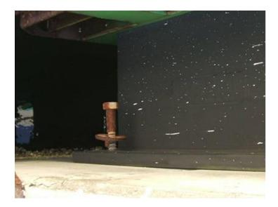
Photo 2.3.9 Loose fixing bolt
