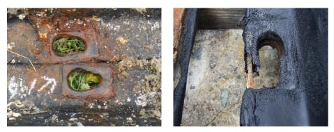
Photo 3.2.1 Re-installation not recommended (Example)
