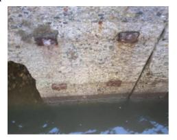
Photo D-1 Example of deterioration rank (Fixings)
