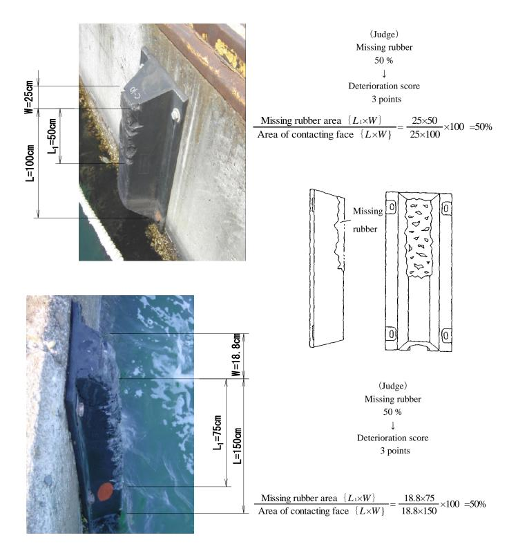
Photo C-4 Example of damage (Missing rubber)
