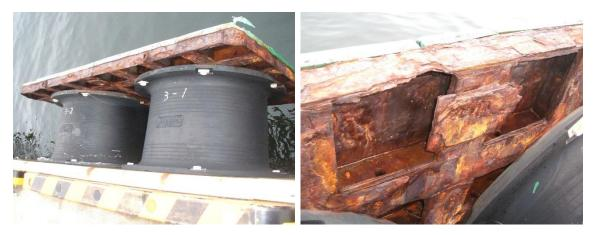
Photo 3.3.1 Example of damage rank "a" of fender panel corrosion
