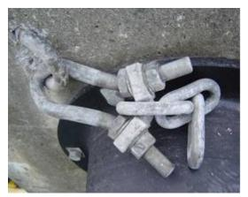
Photo 2.3.14 Bent support (Adjustable U-shape shackle)
