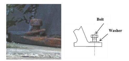
Photo 2.2.12 Loose fixing bolt (Accessories)
