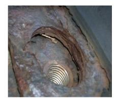
Photo 2.2.14 Missing fixing bolt (Accessories)
