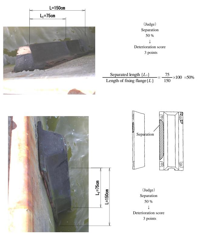
Separated length  $\{L_1\}$ Length of fixing flange  $\{L\}$  =  $\frac{75}{150} \times 100 = 50\%$
