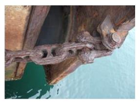
Photo 2.3.16 Corrosion of support (Chain)
