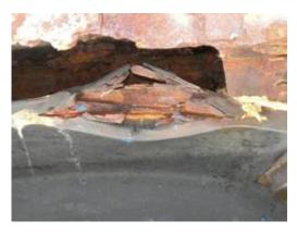
Photo 2.3.4 Separation of rubber body
