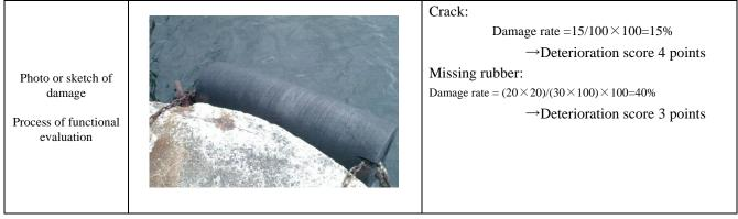
Fig. 3.5.4 Example of check sheet (cylindrical fender)
