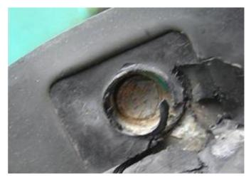
Photo 2.3.12 Cut fixing bolt
