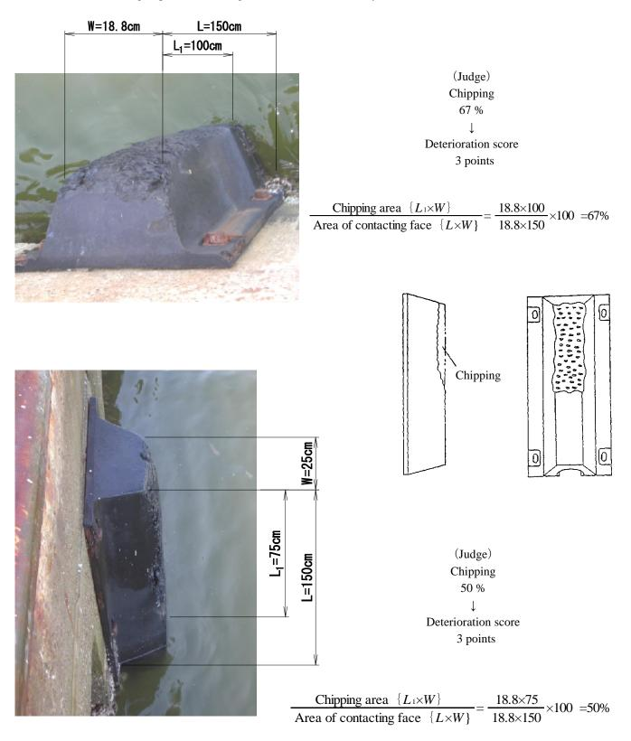
Photo C-6 Example of damage (Chipping)
