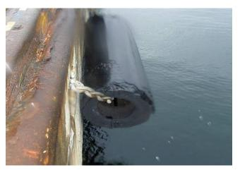
Photo 2.5.2 Missing rubber from rubber body
