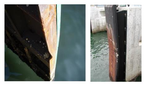
Photo 2.3.7 Deformation of a fender panel
