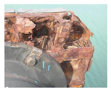
Photo 2.3.8 Corrosion of a fender panel
