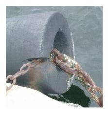
Photo 3.5.2 Example of damage (Cylindrical fender-Tear)
