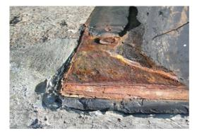
Photo 2.2.15 Cut fixing bolt (Accessories)
