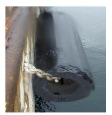
Photo 3.5.1 Example of damage (Cylindrical fender-Missing rubber)
