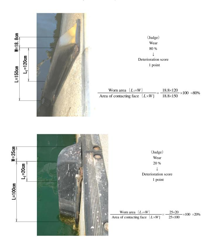
Photo C-8 Example of damage (Wear)
