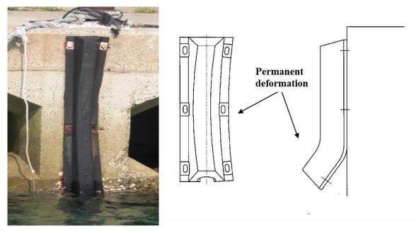
Photo 2.2.3 Permanent deformation of a rubber body
