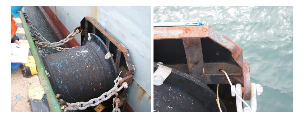
Photo 3.3.2 Example of damage rank "c" of fender panel corrosion
