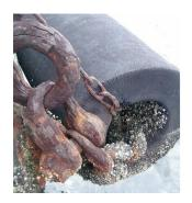
Photo 3.5.3 Example of damage rank "c"
