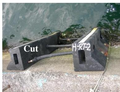
Photo 3.6.1 Example of cut on step of Rubber ladder-Deterioration score “6 point”
