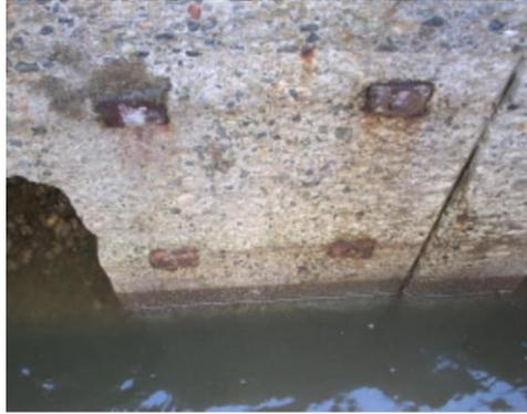
Photo D-1 Example of deterioration rank (Fixings)
