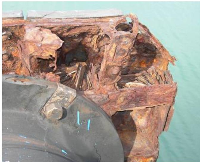
Photo 2.3.8 Corrosion of a fender panel
