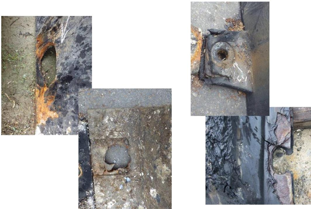
Photo 2.2.11 Bolt hole damage to a rubber body
