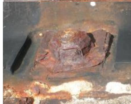
Photo D-2 Example of deterioration rank (Corrosion)
