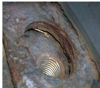
Photo 2.2.14 Missing fixing bolt (Accessories)
