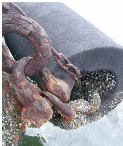
Photo 2.5.4 Corrosion of support
