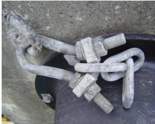
Photo 2.3.14 Bent support (Adjustable U-shape shackle)
