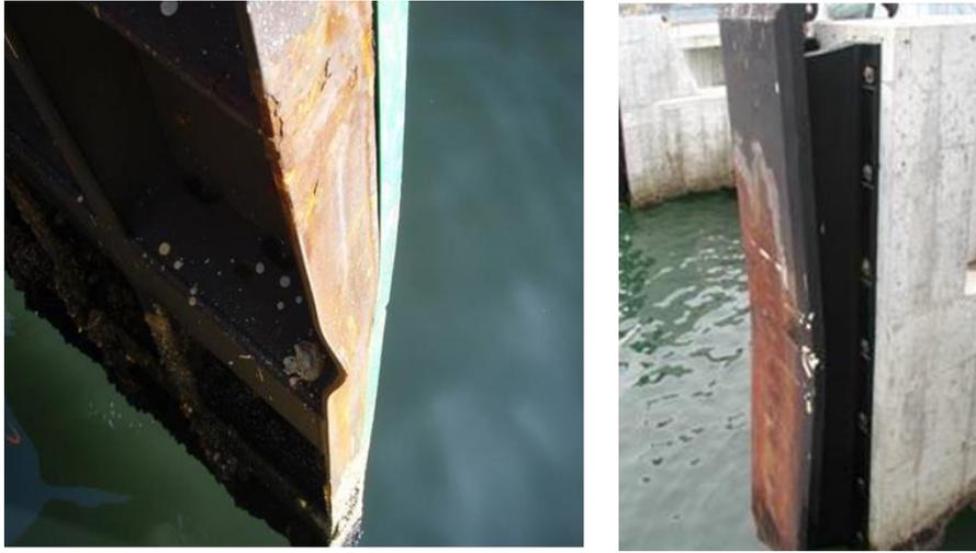
Photo 2.3.7 Deformation of a fender panel
