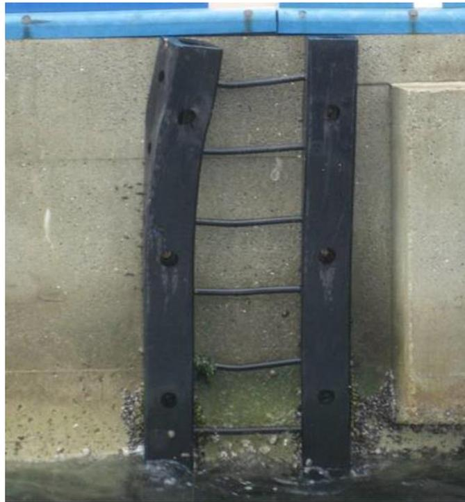
Photo 2.6.3 Permanent deformation of a rubber body
