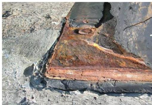
Photo 2.2.15 Cut fixing bolt (Accessories)
