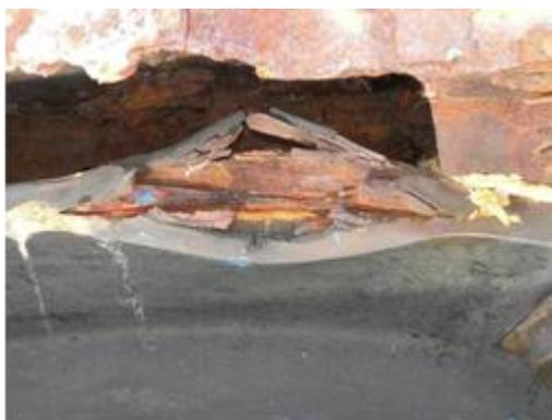
Photo 2.3.4 Separation of rubber body
