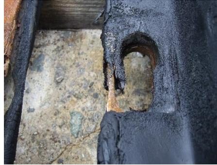
Photo 3.2.1 Re-installation not recommended (Example)
