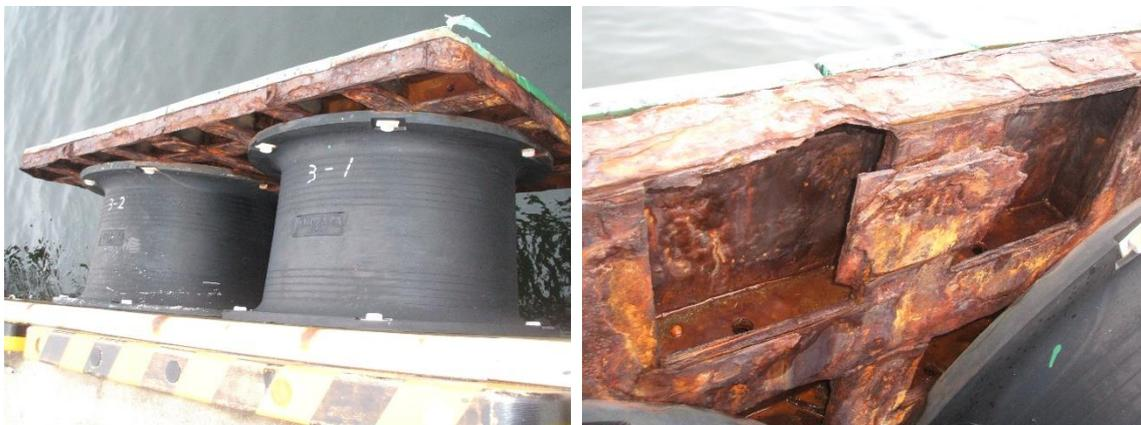
Photo 3.3.1 Example of damage rank “a” of fender panel corrosion
