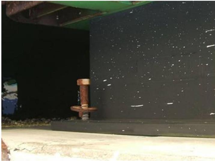
Photo 2.3.9 Loose fixing bolt
