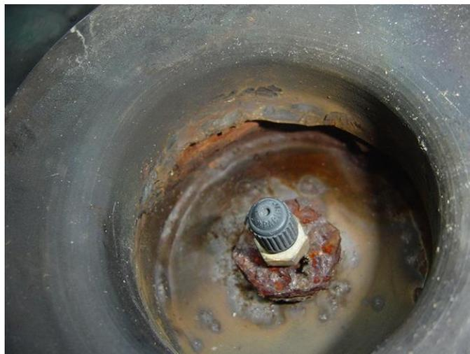
Photo 2.4.2 Separation of rubber body (Embedded plate)
