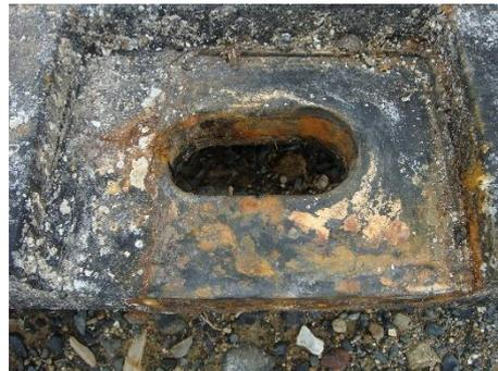
If the coated rubber is peeled off and the iron plate is exposed but there is no decrease in thickness, the failure rate is calculated as separation.
