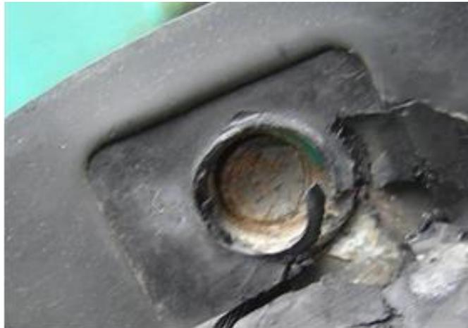
Photo 2.3.12 Cut fixing bolt
