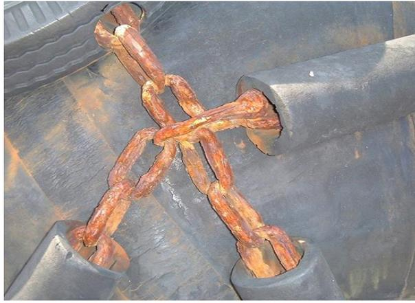
Photo 2.4.11 Corrosion of net
