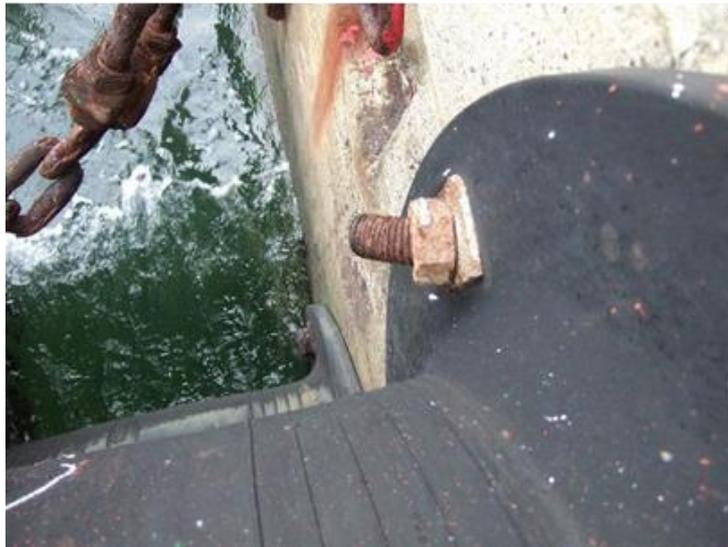
Photo 2.3.10 Bent fixing bolt
