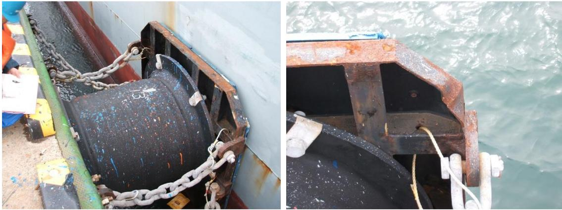
Photo 3.3.2 Example of damage rank “c” of fender panel corrosion
