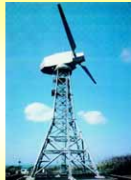
100kW Wind Power Generation System (Miyakejima Tokyo)
