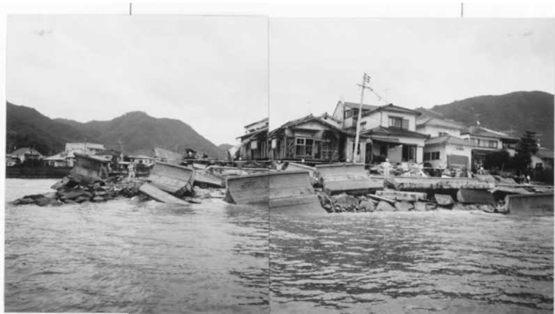
Photo.1 Seawalls and houses damaged by storm surge and waves generated Typhoon 0418 in Kure city
