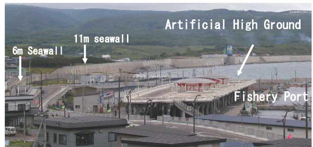
Fig. 11 Completed tsunami mitigation works
