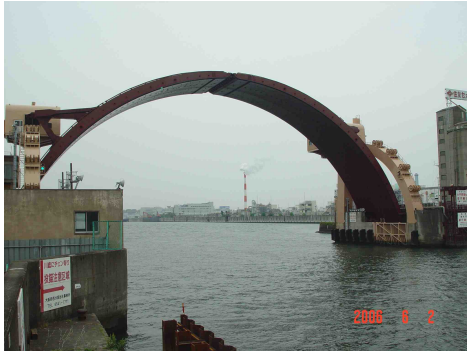
Arch type water gate at Aji River
