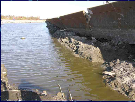
GIWW / MRGO, North Bank (New Orleans East): Overtopped Floodwall (Massive Backscour)
