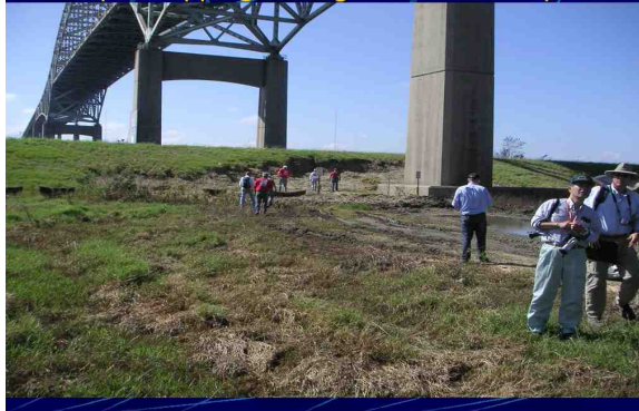
GIVWW / MRGO Levee - Compacted fill (overtopping damage but no failure!)
