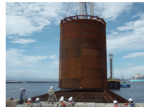
Steel plate cell: Yokohama port
