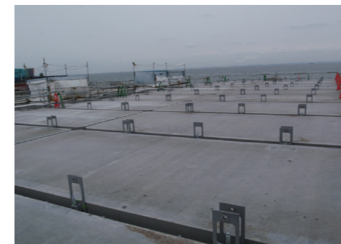
Airport pavement using UFC slab (Ultra high strength Fiber reinforced Concrete: it is light, strong and very durable) (Photo: Haneda D-Runway Expansion JV)
