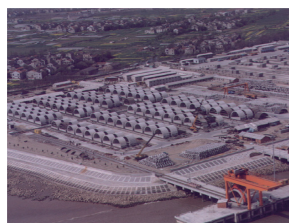
Overseas port facility constructed based on Japanese standards (Semi-circular breakwater: Yangtze River, China)
