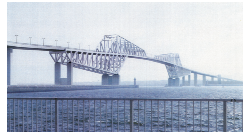
Tokyo Gate Bridge (image after completion) (Photo: Tokyo Port office, Kanto Regional Development Bureau, Ministry of Land, Infrastructure, Transport and Tourism)
