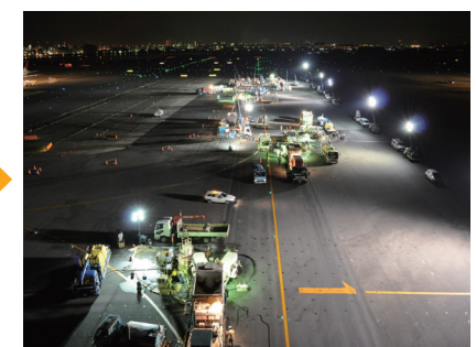
Tokyo International Airport (Haneda Airport) where compaction grouting method was applied for liquefaction countermeasure.
