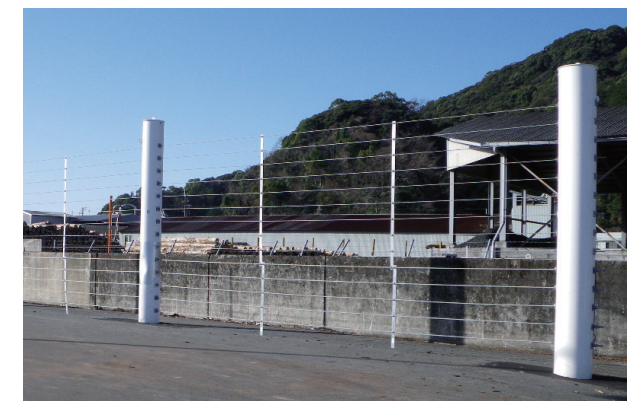
Tsunami driftage capturing facility
