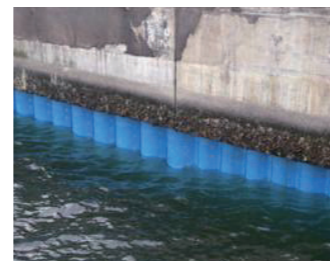
An example of mortar coating method using FRP covering
