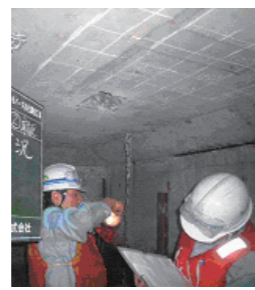
Inspection of Aging condition
