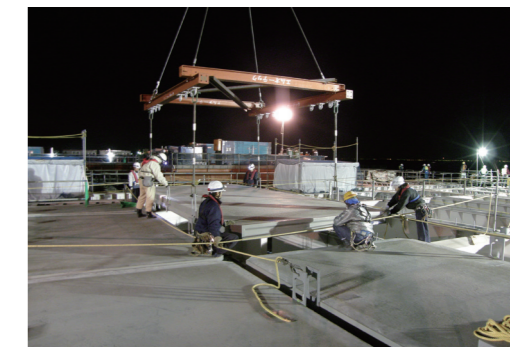
Airport pavement using UFC slab (Ultra high strength Fiber reinforced Concrete: it is light, strong and very durable) (Photo: Haneda D-Runway Expansion JV)
