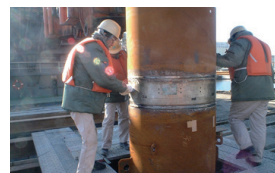
Rakunikan Joint (a mechanical coupler for steel pipe piles or sheet piles to connect each other in a shorter period than a currently used welded joint)
