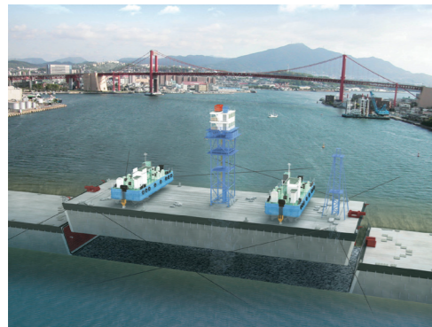
Immersed tunnel installed in New Wakato Harbor Highway
