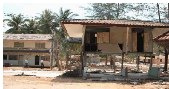
Fig.6 A Wooden House Sustaining Columns in its First Floor
