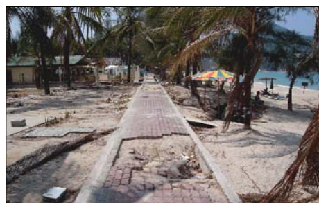
Fig.4 A Pathway Damaged by the Suction of its Base Sand
