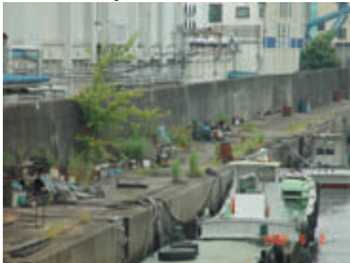
Old sea wall as storm surge barrier
