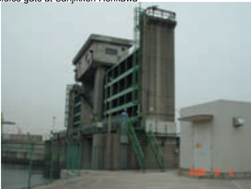
Sluice gate at Sanjikken Horikawa
