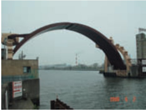
Arch type water gate at Aji River
