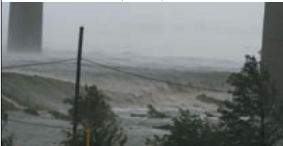
Entergy Levee Overtopping (from their security camera)
