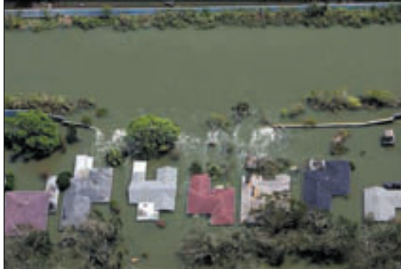
London Avenue Breach at Robert E. Lee Street (425')
