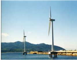
Wind power generation
